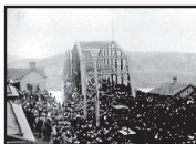
"County Bridge" (now Walnut Street Bridge) on March 19, 1906.
