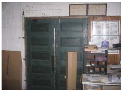
Original Five-Paneled Wood Doors
